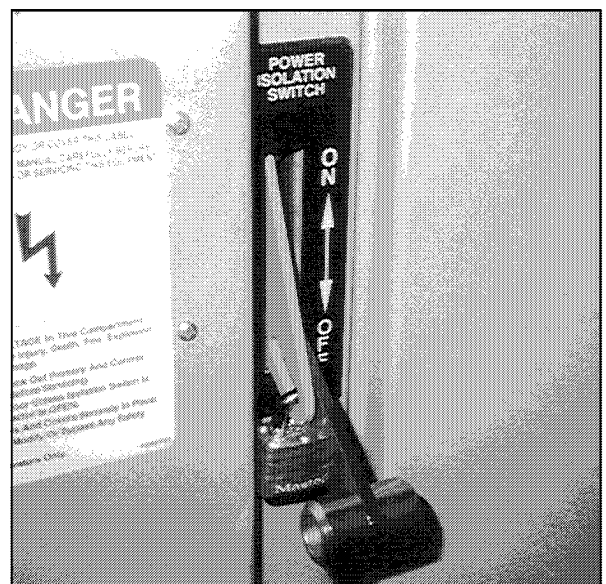
Fig. 9 Isolation Switch Lockout
