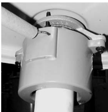
Figure 17. Internal bushing-mounted current transformer.
