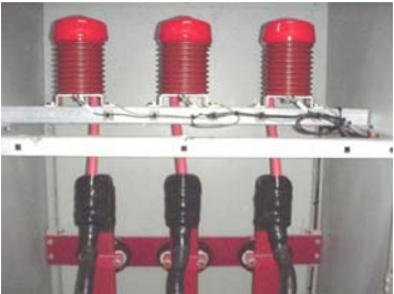
Coupling Capacitor Installation
