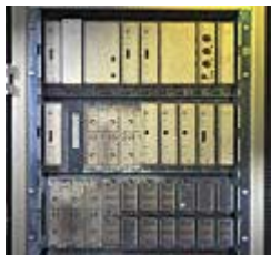
Fig.1 shows one resulting complete 19" 12U tall relay terminal type RAGCX for generator protection built up from modular COMBIFLEX components. Redundancy is achieved through individually operating functional modules and DC supply divided into two separate groups.
