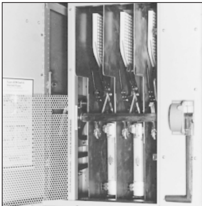
Fig. 1 ADM Switch with Safety Screen Removed
