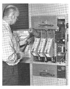
**3** Using the fuse puller, follow the FUSE REMOVAL instructions on the door to pull the arc boxes out and remove the power fuses.
