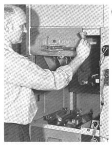
Remove the two socket head cap screws located in the front casting of the isolation switch. SAVE THESE CAP SCREWS.
