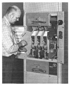
Push the arc boxes back into their normal operating position. Remove the four phase barriers from the contactor by lifting the bottom of barrier slightly and rotating top out toward you.
