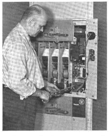
2 Remove the fuse puller from its track alongside the contactor.
