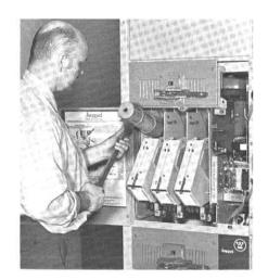
17 Before replacing power fuses, check that fuse clamps are in their proper position. Refer to illustration on starter door. Fuse clamp guide should be in the fuse clamp positioner. Check fuse rating against fuse data on starter door to be sure correct fuses are installed. Install power fuses using fuse puller. Instructions are on starter door. Fuses will be loose in fuse clamps — this is normal. Full clamping pressure is applied when the isolating switch is closed.
