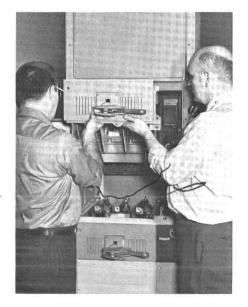
10 Pull the isolation switch toward you on its rails. CAUTION - It has no latch and will pull completely out. However, it weighs only 75 pounds and can be handled by two men.
