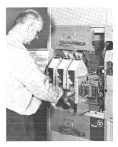
6 Using the front flange of the contactor end frame, pull the contactor free of the rear stab connectors. Carefully pull the contactor out as far as it will go. It will be stopped by a latch about ¾ of the way out. This position is used for contactor maintenance.
