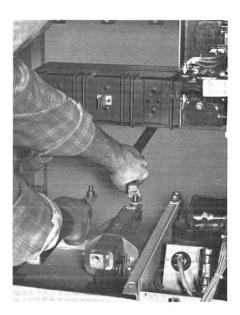
12 Wire to line terminals (top of starter cell) and load terminals (bottom, rear). Connect ground lead to ground connection in bottom lefthand corner of cell.
