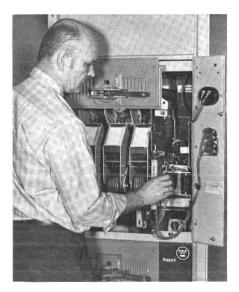
Framework from the Remove the control plug from the right-hand side of the contactor.
