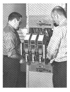
Lift out the contactor. You can use the rectangular holes on the lefthand side and the control plug bracket and main shaft on the right hand side for hand grips.
