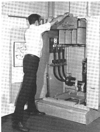
13 Slide isolation switch back in place, and secure with 2 bolts.
