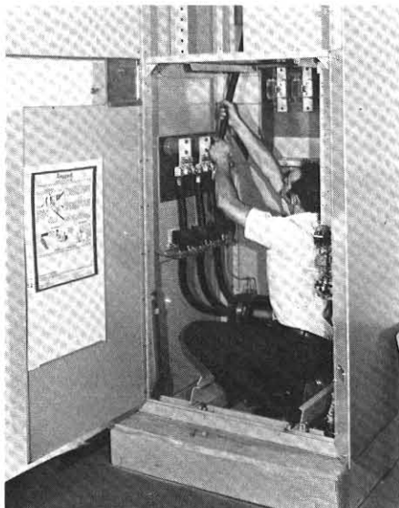
12 Pull cables to starter load terminals. After wiring replace access panels.
