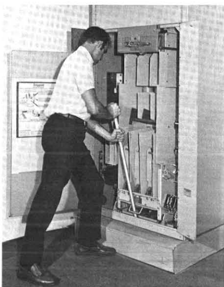
15 Put jiffy bar through the "D" handle and into the channel. Pry contactor onto load stabs.
