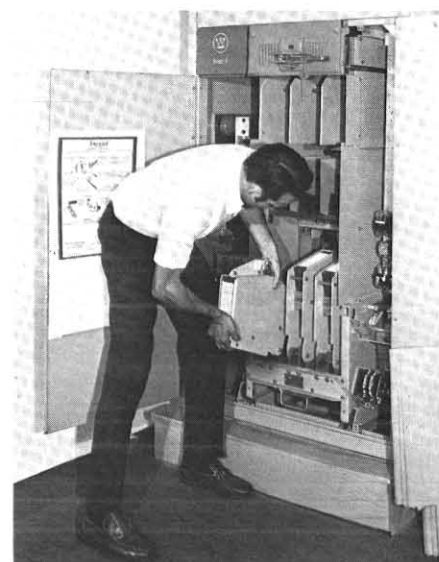
17 Rotate blowout irons forward and down. CAUTION — Make sure the 3 arc boxes and 4 phase barriers are in place. Door will not close if blowout irons are in the wrong position.
