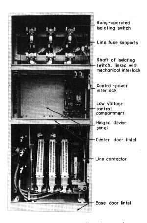
Fig. 2. Typical Limitamp controller showing location of principal components
