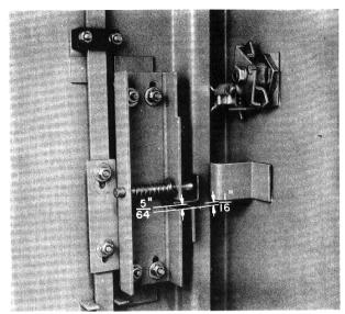
Fig. 6. Close-up view of "door forgetter" interlock adjustment
