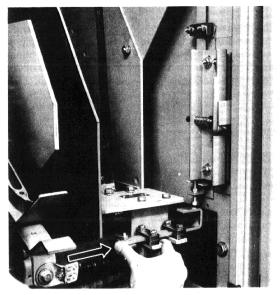
Fig. 11. View showing vertical rod mechanically connected to gang-operated isolating switch; interference interlock prevents vertical rod from being lowered when the contactor is energized. To check freedom of movement of contactor interlock, move horizontal arm to right with one finger at point of arrow. Little force should be required and action should be smooth and positive
