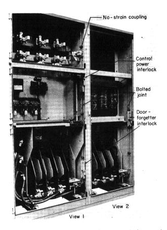
Fig. 5. View 1 shows mechanical door interlock as used on basic panels containing isolating switches; view 2 shows additional interlocking arrangement used when panel has one or more sections of high-voltage components connected to the load side of the isolating switch
