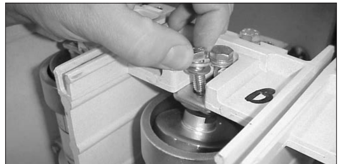
Figure 19. Remove Bolt Securing Vacuum Interrupter
