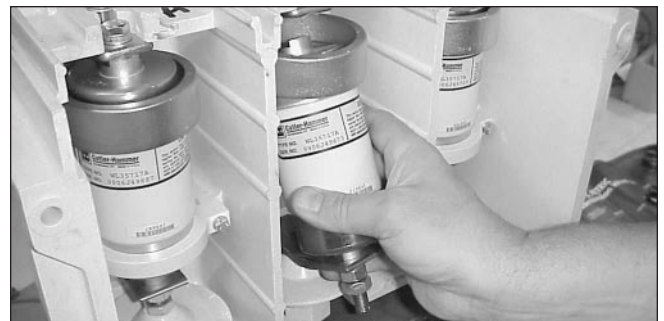
Figure 20. Hold Insulator Down
