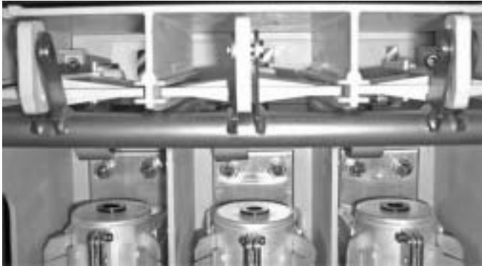
View of Isolation Switch Through Viewing Window
