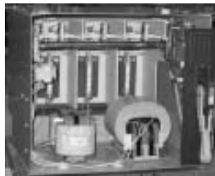
Potential Transformers, Control Power Transformer and Fuses Mounted in a disconnect assembly, Height 20 Inches (508 mm)
