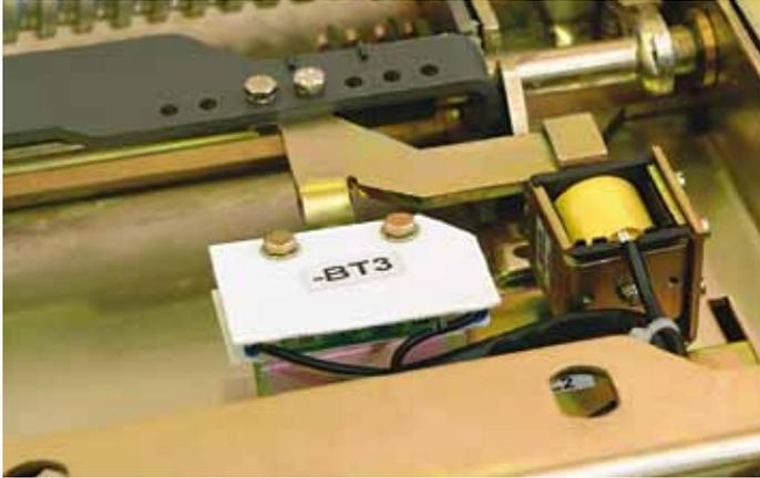
This only allows the withdrawable contactor to be racked into/out of the enclosure with the electromagnet energised and the contactor open.
