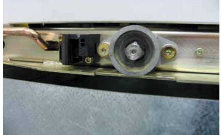
Isolation lock for UniGear switchgear and PowerCube modules. It prevents the apparatus from being racked-in if the unit door is open.
