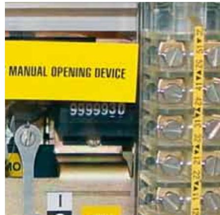
Mechanical operation counter for fixed versions, electric impulse operation counter for withdrawable versions. This is a device which counts the contactor closing cycles.
