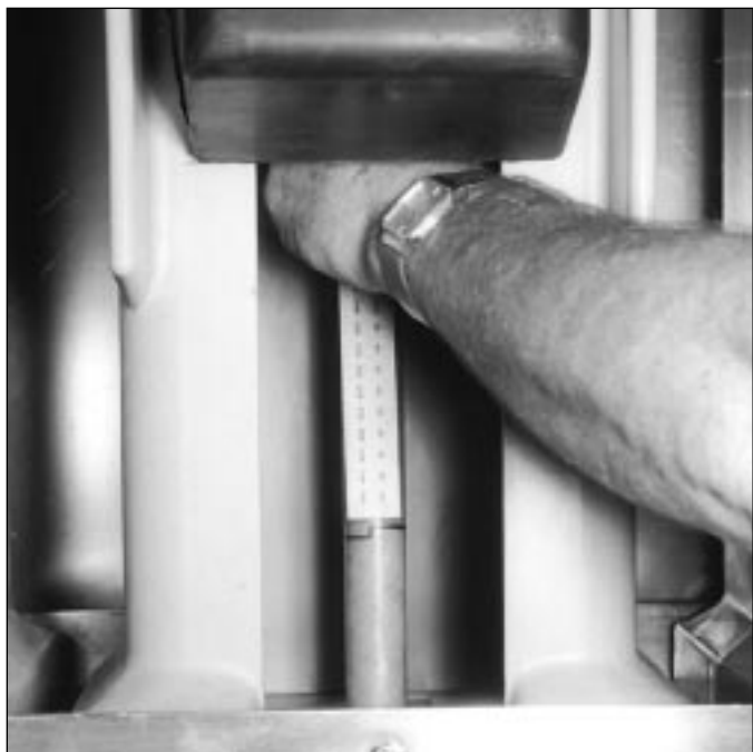
Figure 6-2 Rear Measurement for Contact Erosion Being Made (Circuit Breaker Closed)
