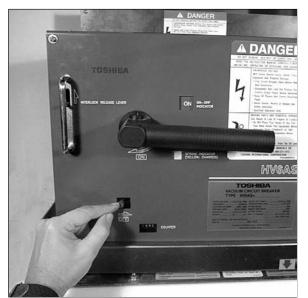
Fig. 27 Manually Opening Breaker
