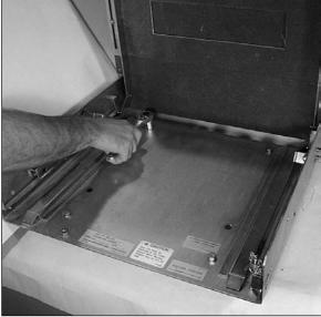
Fig. 11 Fastening Cell to Compartment Floor or Shelf
