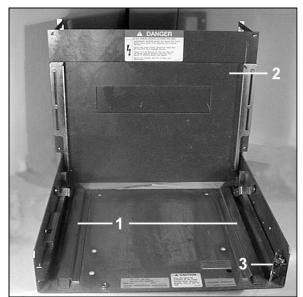
Fig. 2 Type H6A-HLS Circuit Breaker Cell
