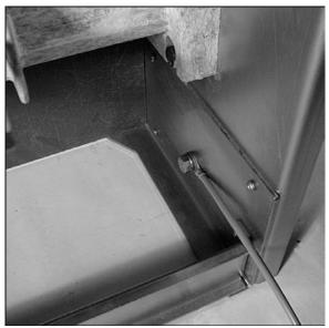
Fig. 14 Installation of Ground Wire
