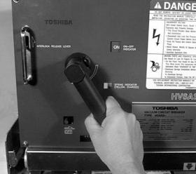
Fig. 26 Manually Closing Breaker
