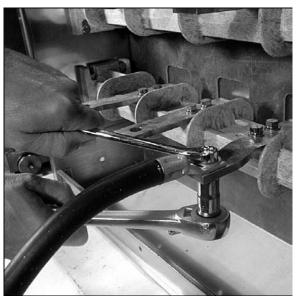
Fig. 12 Fastening Cables to Main Circuit Terminals
