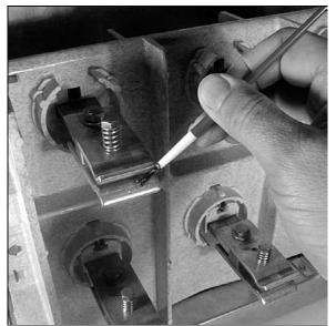
Fig. 17 Apply B9 Grease to Stab Fingers
