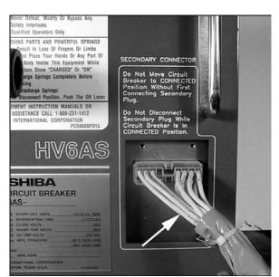
Fig. 16 Control Wire Harness
