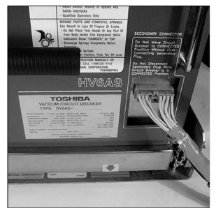
Fig. 23 Breaker at DISCONNECTED Position
