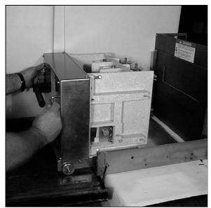
Fig. 19 Inserting Breaker into Cell
