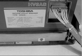
Fig. 21 Control Circuit Plug Connected to Breaker
