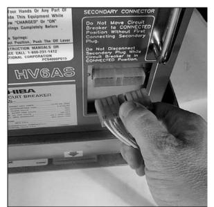
Fig. 24 Disconnect Control Circuit Plug
