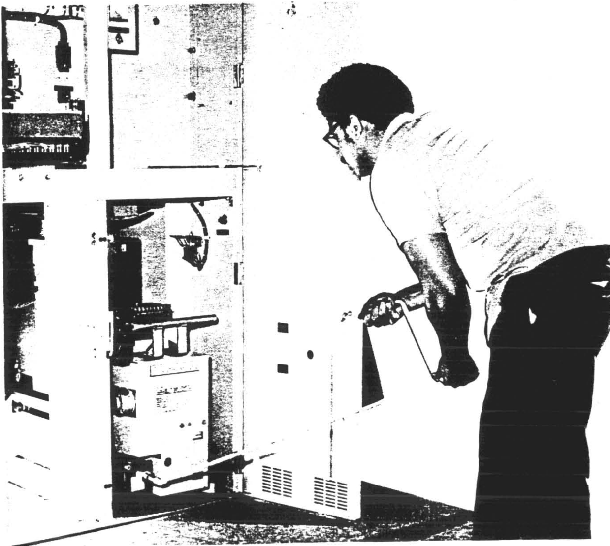
Figure 38. Breaker Racking, Manual
