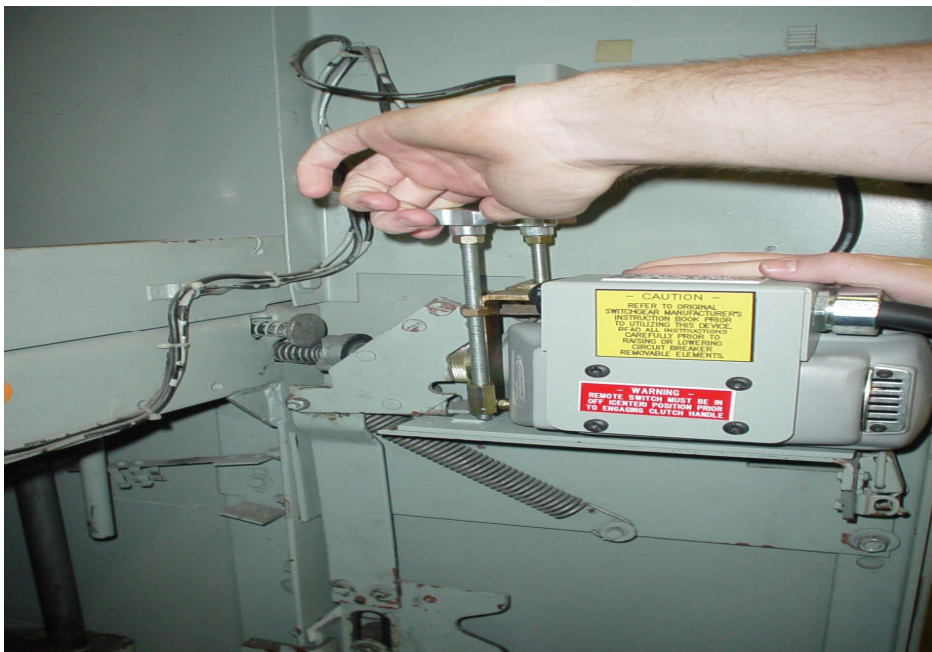
Figure 5 – Locking Hinge Assembly in Place
