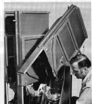
Tilting the arc chutes. Released for easy tilting. One
