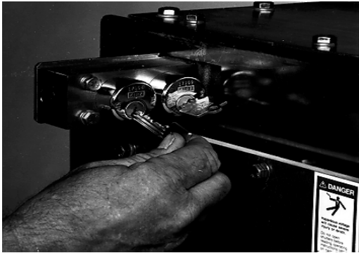
FIGURE 3.2.1 INSERT KEY KU IN KEY LOCK K1 AND ROTATE
