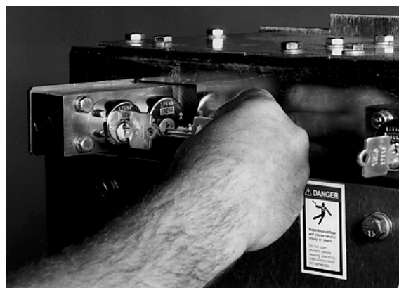
FIGURE 3.5.7 ROTATE KEY KU AND REMOVE KEY KB FROM KEY LOCK K1
