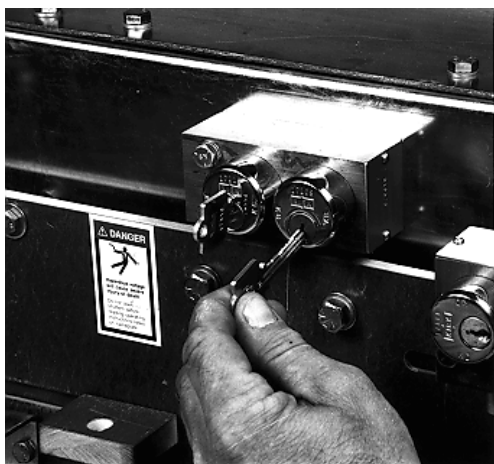
FIGURE 3.3.9 INSERT KEY KB IN KEY LOCK K2 AND ROTATE KEY KC
