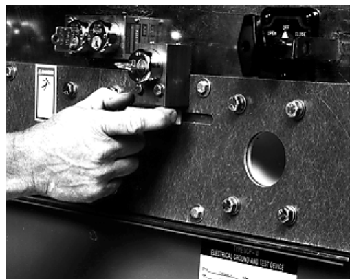
FIGURE 3.5.11 INSERT KEY KD IN KEY LOCK K5 AND ROTATE, REMOVE PROBES
