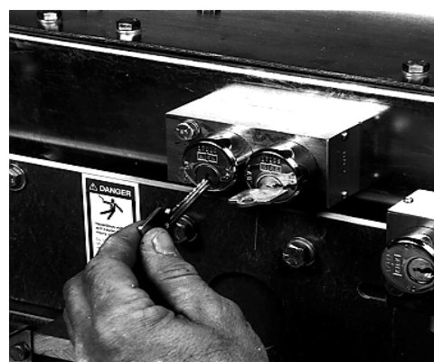
FIGURE 3.2.12 INSERT KEY KC IN KEY LOCK K2 AND ROTATE.
