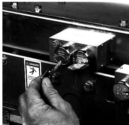
FIGURE 3.5.20 ROTATE KEY KU AND REMOVE KEY KB FROM KEY LOCK K1
