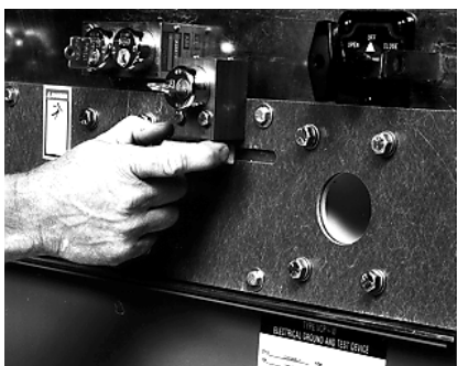
FIGURE 3.4.25 OPEN TEST PORT SHUTTER
