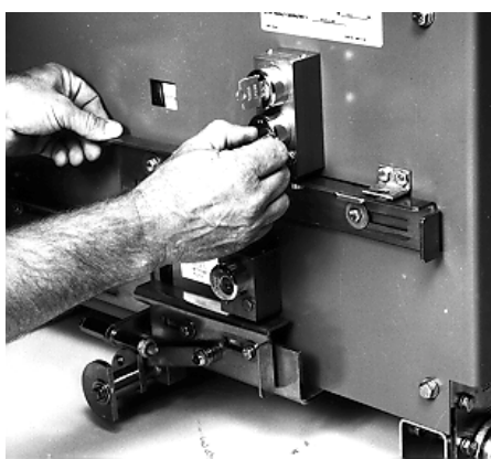
FIGURE 3.4.28 INSERT KEY KD IN KEY LOCK K4 AND ROTATE
