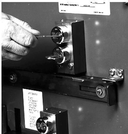
FIGURE 3.4.29 REMOVE KEY KB FROM KEY LOCK K4
