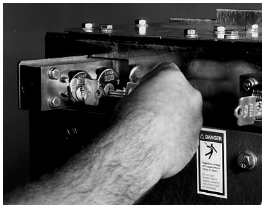
FIGURE 3.5.1 INSERT KEY KB IN KEY LOCK K1 AND ROTATE KEY KU
