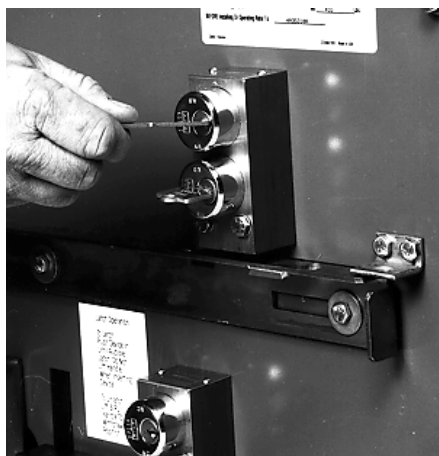
FIGURE 3.4.21 INSERT KEY KB IN KEY LOCK K4
