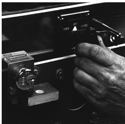
FIGURE 3.4.19 TURN SELECTOR SWITCH TO "OFF" POSITION
