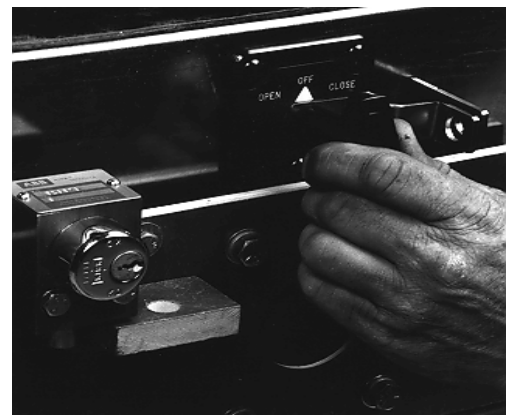
FIGURE 3.3.6 TURN SELECTOR SWITCH TO "OFF" POSITION
