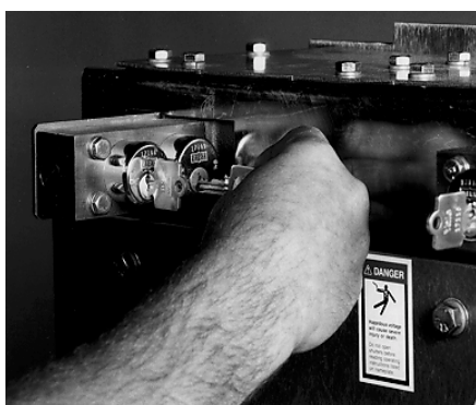
FIGURE 3.4.35 ROTATE KEY KU AND REMOVE KEY KB FROM KEY LOCK K1
