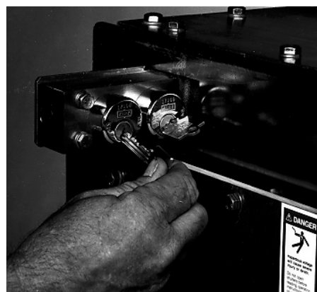
FIGURE 3.3.18 REMOVE KEY KU FROM KEY LOCK K1
