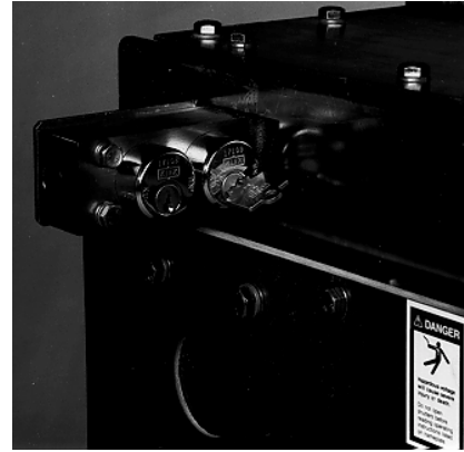
FIGURE 2.3.1 KEY LOCK K1 INTERLOCK
