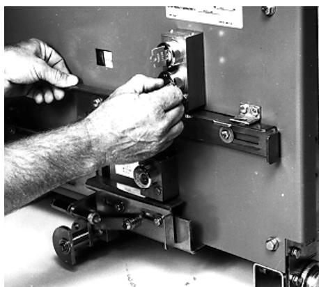
FIGURE 3.4.23 REMOVE KEY KD FROM KEY LOCK K4
