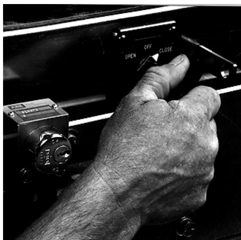
FIGURE 3.4.17 TURN SELECTOR SWITCH TO "CLOSE" POSITION
