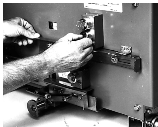
FIGURE 3.5.10 REMOVE KEY KD FROM KEY LOCK K4
