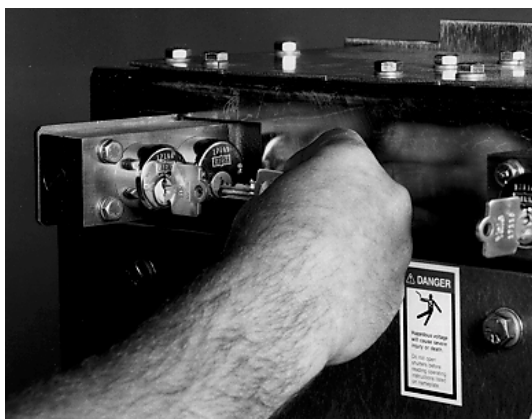
FIGURE 3.2.21 ROTATE KEY KU AND REMOVE KEY KB FROM KEY LOCK KI
