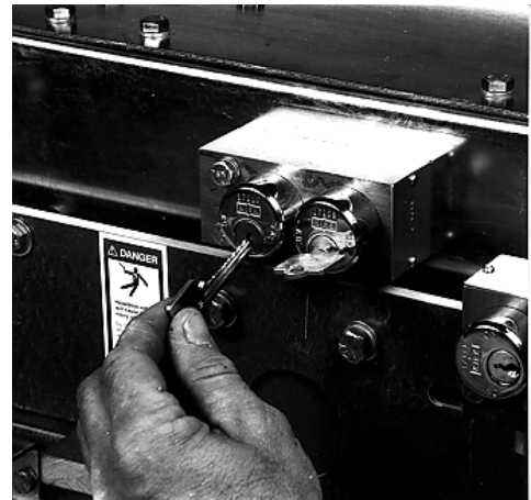
FIGURE 3.4.4 REMOVE KEY KC FROM KEY LOCK K2
