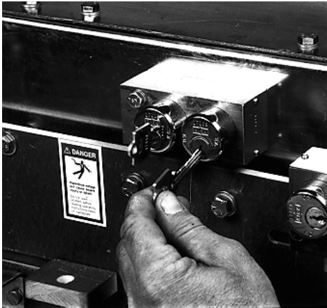
FIGURE 3.4.3 I INSERT KEY KB IN KEY LOCK K2 AND ROTATE KEY KC
