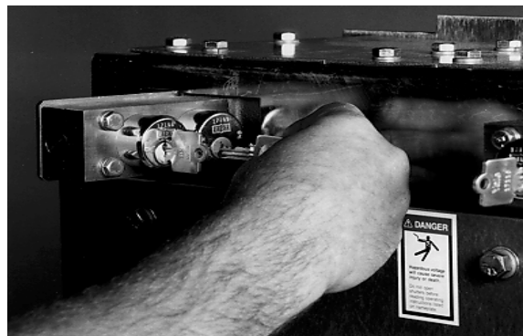
FIGURE 3.3.8 ROTATE KEY KU AND REMOVE KEY KB FROM KEY LOCK K1
