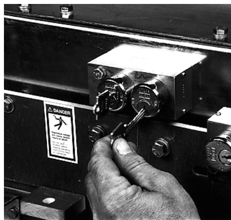
FIGURE 3.3.16 REMOVE KEY KB FROM KEY LOCK K2
