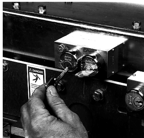
FIGURE 3.4.12 INSERT KEY KC IN KEY LOCK K2 AND ROTATE
