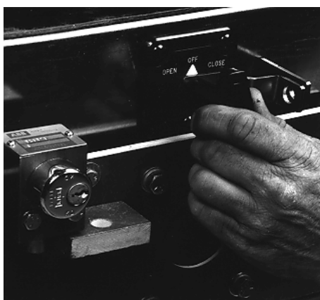
FIGURE 3.4.33 TURN SELECTOR TO "OFF" POSITION
