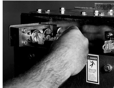
FIGURE 3.2.2 REMOVE KEY KB FROM LOCK K1
