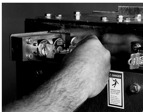
FIGURE 3.3.17 INSERT KEY KB IN KEY LOCK K1 AND ROTATE KEY KU
