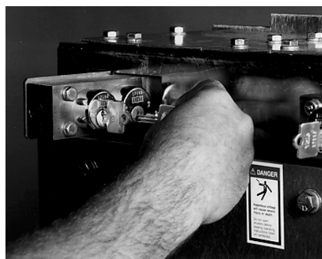
FIGURE 3.4.14 INSERT KEY KB IN KEY LOCK K1 AND ROTATE KEY KU.
