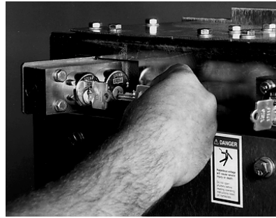
FIGURE 3.2.14 INSERT KEY KB IN KEY LOCK K1 AND ROTATE KEY KU
