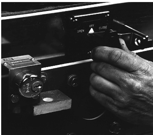
FIGURE 3.2.19 TURN SELECTOR SWITCH TO "OFF" POSITION
