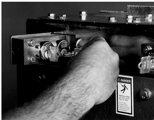
FIGURE 3.5.15 INSERT KEY KB IN KEY LOCK K1 AND ROTATE KEY KU
