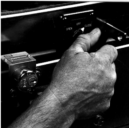
FIGURE 3.2.17 TURN SELECTOR SWITCH TO "CLOSE" POSITION
