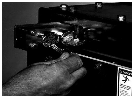
FIGURE 3.5.30 REMOVE KEY KU FROM KEY LOCK K1
