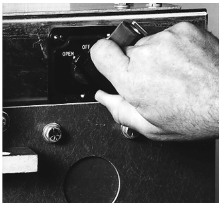
FIGURE 3.4.31 TURN SELECTOR SWITCH TO "OPEN" POSITIONS
