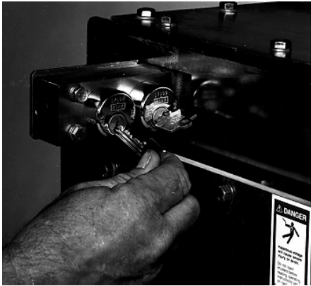
FIGURE 3.4.1 INSERT KEY KU IN KEY LOCK K1 AND ROTATE
