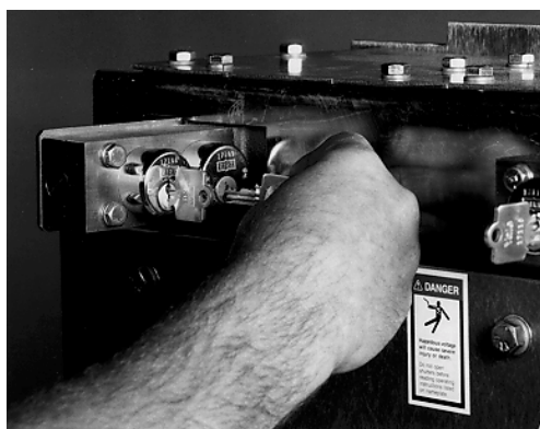
FIGURE 3.5.29 INSERT KEY KB IN KEY LOCK K1 AND ROTATE KEY KU
