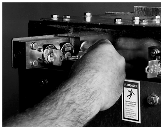
FIGURE 3.4.20 ROTATE KEY KU AND REMOVE KEY KB FROM KEY LOCK K1
