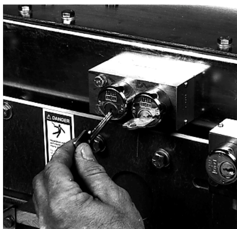
FIGURE 3.5.27 INSERT KEY KC IN KEY LOCK K2 AND ROTATE
