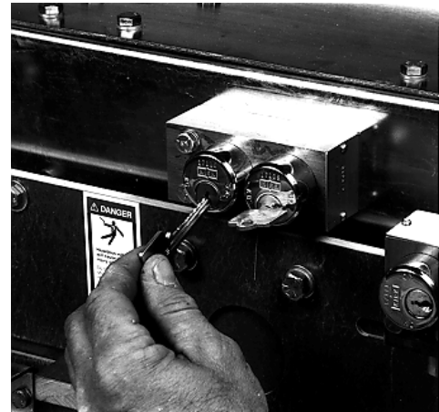
FIGURE 3.2.4 REMOVE KEY KC FROM KEY LOCK K2
