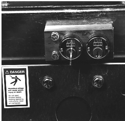
FIGURE 2.3.2 KEY LOCK K2 INTERLOCK
