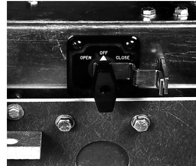
FIGURE 3.3.2 VERIFY THAT THE SELECTOR SWITCH IS IN THE "OFF" POSITION.
