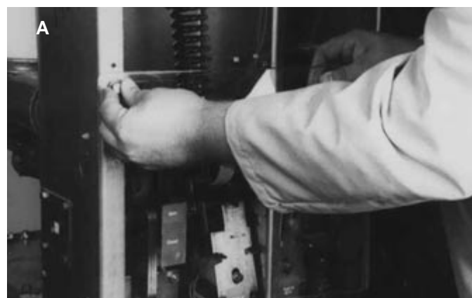
Figure 6-9 Attaching CloSure™ Test Tool at Hole “A”
