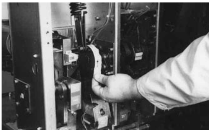
Figure 6-16 Remove Marked Masking Tape from Cam
