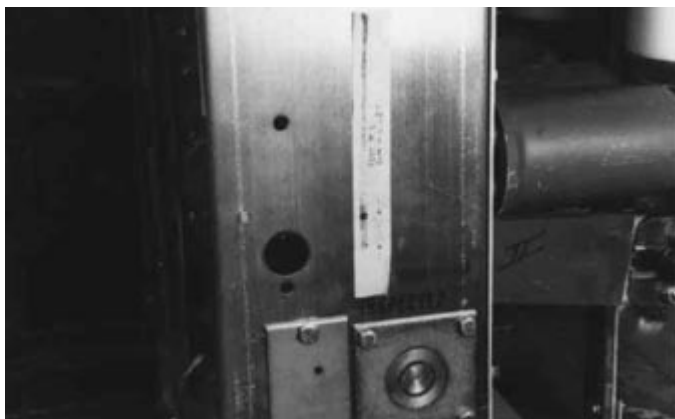
Figure 6-17 Place Tape on Right Side Panel of Breaker
