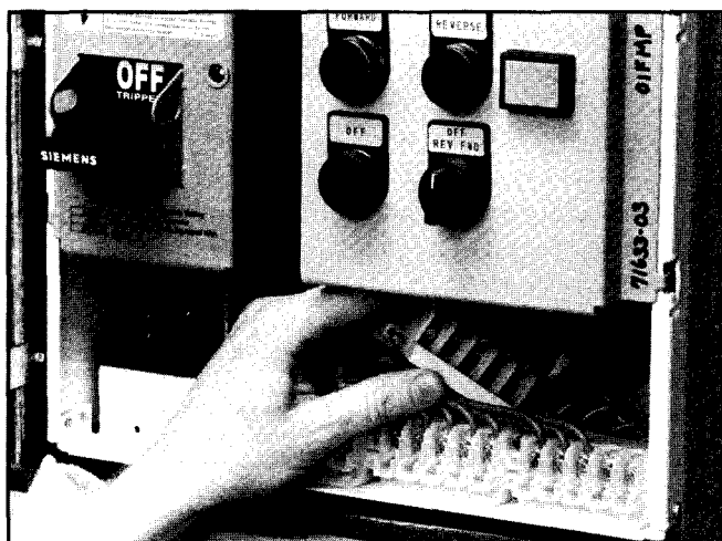
Figure 21B. Moving Terminal Blocks into the Wireway
