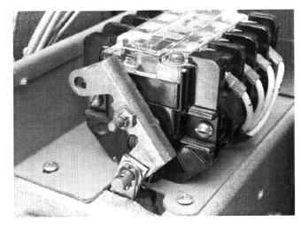
Working from the bottom of the Breaker, align the holes in the Drive Link and the Reset Rod Assembly with the hole in the Pull Shaft Stop as shown. It may be necessary to slightly compress the spring on the Reset Rod to achieve proper alignment.
