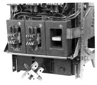
A. Drill one .219" diameter hole in each side of the rear Breaker Frame (See Drilling Plan "C").
