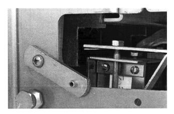
D. Mount the DTA Assembly on the inside of the bottom Breaker Flanges using the holes just drilled and the (2) .250-20 × .750" bolts, (4) flat washers, (2) lock washers, and (2) nuts supplied.
