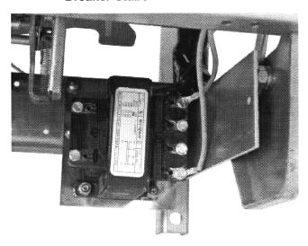
A. Position the fuses in an accessible location then mark and cut the Load Side of each High Voltage Fused Wire (HV Wire). Strip .250" from each Load Side HV Wire and attach a .138" ring terminal to each. Attach the HV Wires to the CPT terminals to achieve the required voltage. (See the following Table.)
