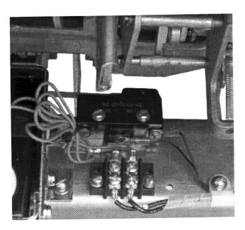
E. For Kits Supplied with a Breaker Mounted CPT Only. Remove the External Harness plug installed in the bottom rear socket on the right side of the Trip Unit. Insert the black plug of the CPT Harness into the same socket. Reinsert the External Harness plug just removed into the female receptacle on the CPT Harness.
