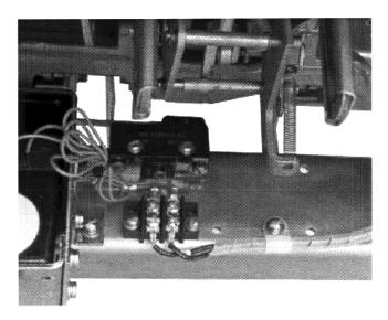
H. Use the nylon wire ties provided to dress all wires and harnesses to keep them away from any moving parts within the Breaker.
