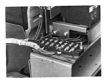
D. Route the Sensor Harness towards the left rear of the Breaker, then through the hole drilled in Step 12-A.
