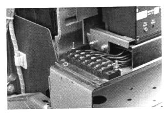
C. Connect the Sensor Harness to the proper terminals of the 7-Point Terminal Block. Refer to Section 12 of the Retrofit Application Data, supplied with the Retrofit Kit, for detailed wiring specifications.
