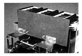
D. Mount the Trip Unit to the Trip Unit Mounting Brackets, as shown, using the (2) brass spacers, (2) .190-32 × 4.00" screws, (2) lock washers, and (2) flat washers.
