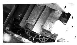
Use the nylon wire ties supplied to dress all wires to keep them away from any moving parts within the Breaker.
