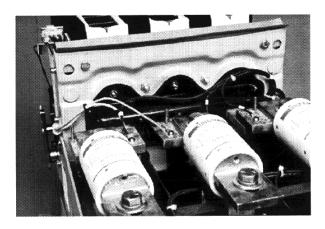
NOTE: The power convention of the Circuit Breakers is normally Top to Bottom, meaning the Top Breaker Stabs are on the Line Side of the Breaker and the Bottom Breaker Stabs are on the Load Side.
