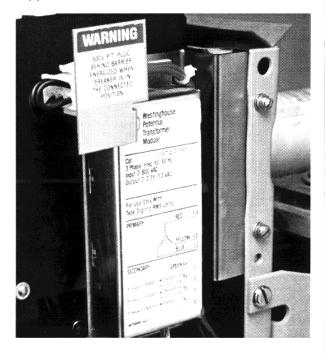
For Kits Supplied with a Breaker Mounted CPT Only. Secure the HV Wires to the Breaker using the wire clamp supplied and the top screw, lock washer, and flat washer mounting the PT Module assembly to the right rear Breaker Frame.
