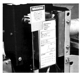
A. Using Drilling Plan C, drill one .203" diameter hole in the right side of the rear Breaker Frame.
