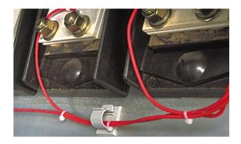
G. Remove the protective cover from the adhesive pad on the back of the Self-Adhesive Wire Clamp. Secure the Clamp to the Breaker Back Plate with the Clamp opening facing upward. Route PT Wires through the Clamp as shown.
