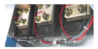
P. Attach the appropriate label for the Breaker in a clearly visible position. Four (4) labels are included with the CPT, one (1) for 600 Volt, one (1) for 480 Volt, one (1) for 240 Volt, and one (1) for 208 Volt systems.
