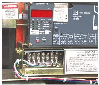
A. Feed the Sensor Harness through the grommet in the left side of the Aux. CT Module. Connect the Sensor Harness to the proper terminals of the Aux. CT Module. Refer to Section 12 of the Retrofit Application Data, supplied with the Retrofit Kit, for detailed wiring specifications.
