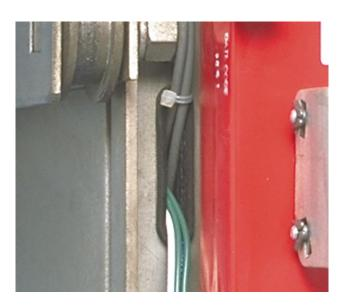
NOTE: The Line Side HV Wires are longer than necessary and are cut during the following steps. Before cutting the wires, be sure that sufficient length is left so that the HV Wire Fuses are accessible from the front of the Breaker and that the connections can be made to the correct Breaker Stabs.
