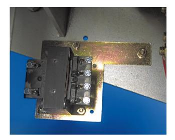
E. The CPT Harness will connect the CPT to the Trip Unit. Temporarily position the plug-in connector of the CPT Harness near the right side of the Trip Unit. Route the CPT Harness down along the inside of the right Breaker frame, then across the bottom of the Breaker, past the Copper Connectors, then to the CPT Assembly.
