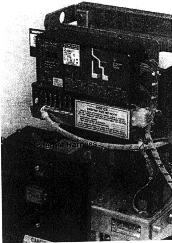
A. Plug the External Harness into the sockets on the right side of the Trip Unit.
