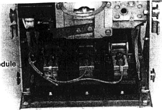
Ring Terminal on each. Attach the wires to the correct .500-13 bolt of each phase with a nut, flat washer and lockwasher left from Step 3A.
