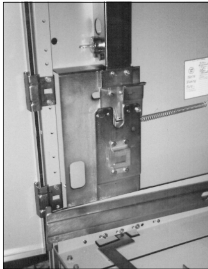
Key Interlock and Linkage
