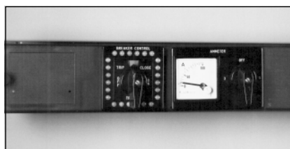
Breaker Control Switch, Ammeter and Switch
