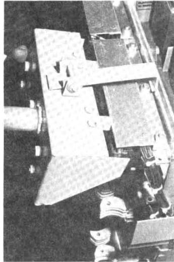
2. Engage the two extended pins of the probe in the slots provided in the secondary contact blocks.
