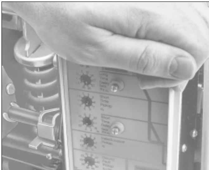
7. Lower trip unit onto support plate.
