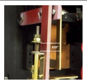
B. Measure the gap between the flat surface of the flange nut on the top of the DTA Shaft and the bottom surface of the Trip Arm. The gap should be .09 to .12". If the gap is not within this range, back off the flange nut and apply Loc-Tite<sup>®</sup> 242 to the threads of the DTA Shaft. Adjust the flange nut until the gap is within the acceptable range.
