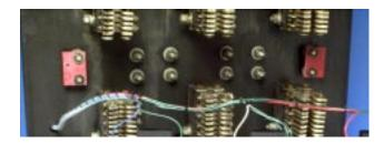
F. With the Sensor Assembly resting on the work surface, close to the Breaker, connect the ring terminals of the Sensor Harness to the Sensors. Refer to Section 12 of the Retrofit Application Data, supplied with the Retrofit Kit, for detailed wiring specifications.
