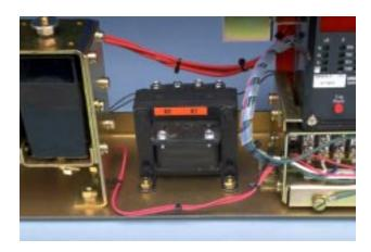
B. Remove the External Harness Plug installed in the Trip Unit. Insert the black plug of the CPT Harness into the same receptacle in the Trip Unit. Reinsert the External Harness Plug just removed into the female receptacle on the CPT Harness.
