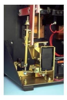
NOTE: Final adjustments to the Reset and Trip Assemblies are performed with the Breaker in the OPEN position.
