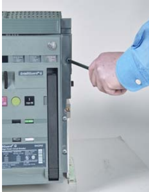
Figure 10. Trip Unit Removal Sequence, Step A
