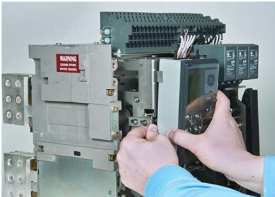
Figure 11. Trip Unit Removal Sequence, Step B
