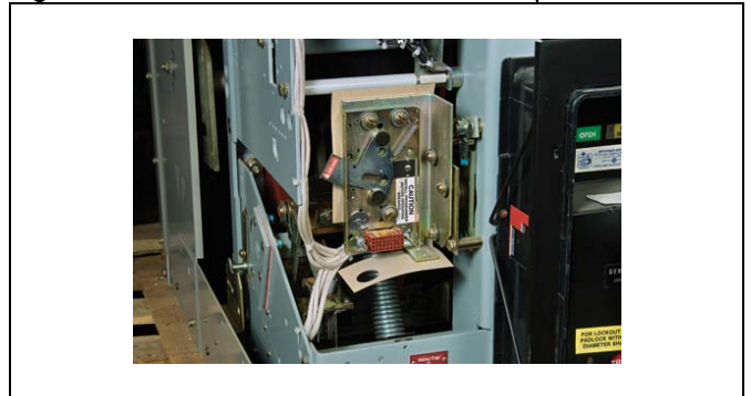
Figure 8: AKR Circuit Breaker without Trip Unit
