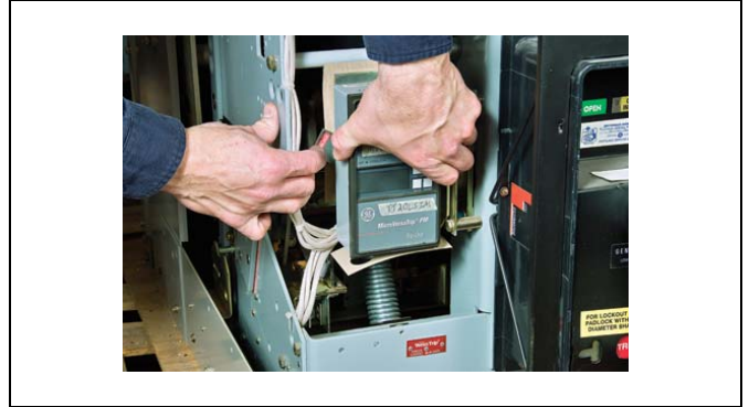
Figure 7: Removing the Old Trip Unit
