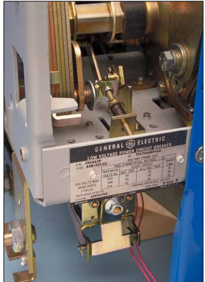
Fig. 17 Reset Link Installed in the Breaker.
