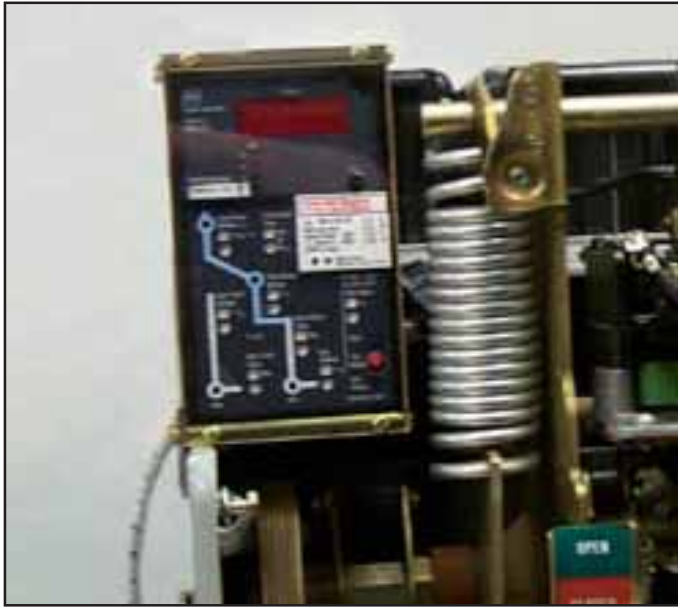
Fig. 22 Overview: Trip Unit Installed on the Breaker.
