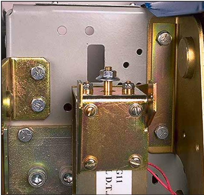
Fig. 15 DTA Assembly Mounted to the Breaker Shelf.
