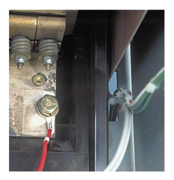
NOTE: The Line Side HV Wires are longer than necessary and are cut during the following steps. Before cutting the wires, be sure that sufficient length is left so that the HV Wire Fuses are accessible from the front of the Breaker and that the connections can be made to the correct Breaker Stabs.
