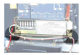
O. Secure the Sensor Harness to the Breaker Platform, as shown, using (1) nylon wire clamp, (1) 164-32 x .500" screw, (2) flat washers, (1) lock washer, and (1) nut.
