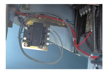
Step 9: Installing the Breaker Mounted CPT
