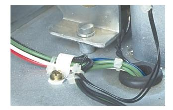
P. Secure the Sensor Harness to the inside of the Breaker Frame with a Wire Clamp, as shown, using (1) nylon wire clamp, (1) 164-32 x .500" screw, (2) flat washers, (1) lock washer, and (1) nut.
