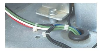
F. Continue to route the Sensor Harness underneath the Breaker Platform to the right side of the Breaker Frame, then through the slotted hole in the right rear of the Breaker Frame as shown. The Sensor Harness will be connected later in the retrofitting process.
