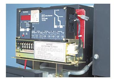
A. Using Drilling Plan "B", drill and tap two (2) .250-20" holes on each side of the Breaker Mechanism. Insure that no drill shavings fall into the Breaker.
