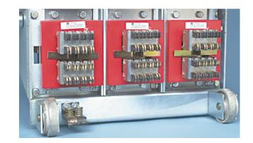
E. Connect the Ring Terminals of the Sensor Harness to the Sensors as shown. Refer to Section 12 of the Retrofit Application Data, supplied with the Retrofit Kit, for detailed wiring specifications.
