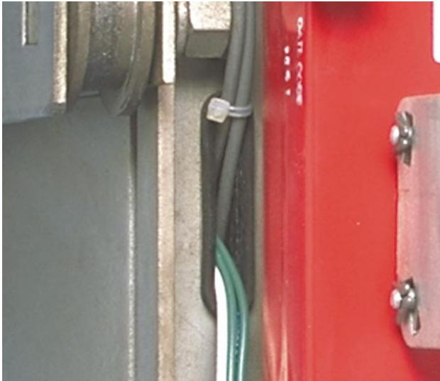
**NOTE:** The Line Side HV Wires are longer than necessary and are cut during the following steps. Before cutting the wires, be sure that sufficient length is left so that the HV Wire Fuses are accessible from the front of the Breaker and that the connections can be made to the correct Breaker Stabs.
