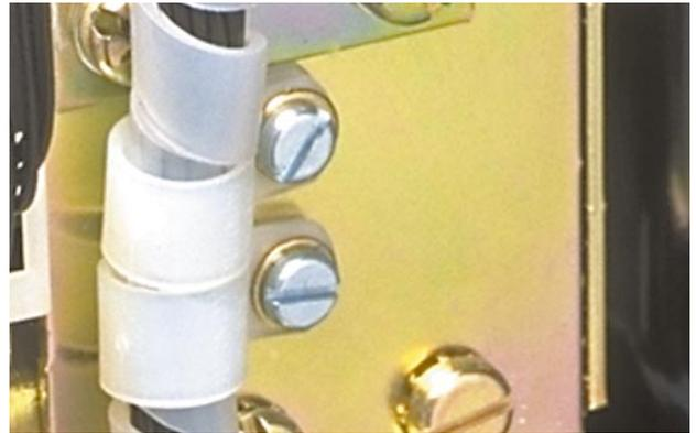
D. *For Kits Supplied with an Auxiliary Switch Only.* Connect the External Harness to the Aux. Switch by routing the two (2) wires (with ring terminals) from the External Harness, along the right Breaker Frame, down to the DTA Assembly. Connect one wire to the normally "Open" terminal of the Aux. Switch and the other wire to the "Common" terminal.
