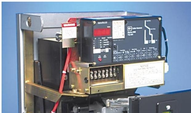
**Step 7: Connecting Sensor Harness and DTA Wires to the Aux. CT Module**
