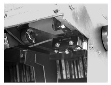
D. Using the .164-32 × .500" screws, flat washers, lock washers, and nuts provided, mount the Aux. Switch Assembly to the right Breaker Frame.
