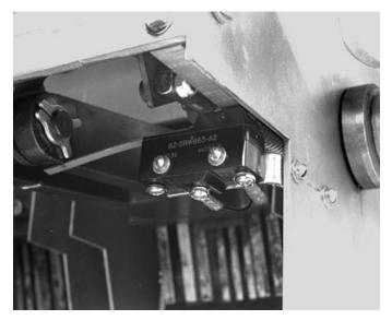
H. Use the nylon wire ties provided to dress all wiring to keep it away from any moving parts within the Breaker.
