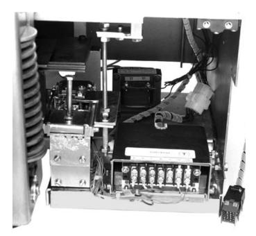
C. Route the Sensor Harness between the Aux. CT Module and the DTA Assembly, out the back of the Breaker, then up to the Sensors. D. Connect the ring terminals of the Sensor Harness to the Sensors. Refer to Section 12 of the Retrofit Application Data, supplied with the Retrofit Kit, for detailed wiring specifications.
