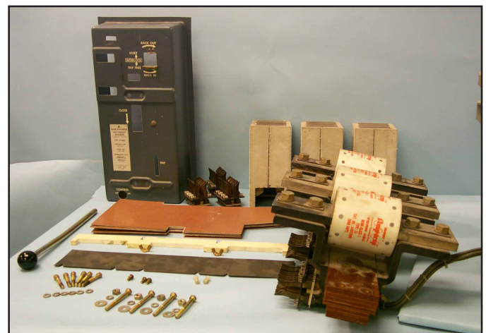
Fig. 2 Original Components Removed and Saved for Reinstallation.
