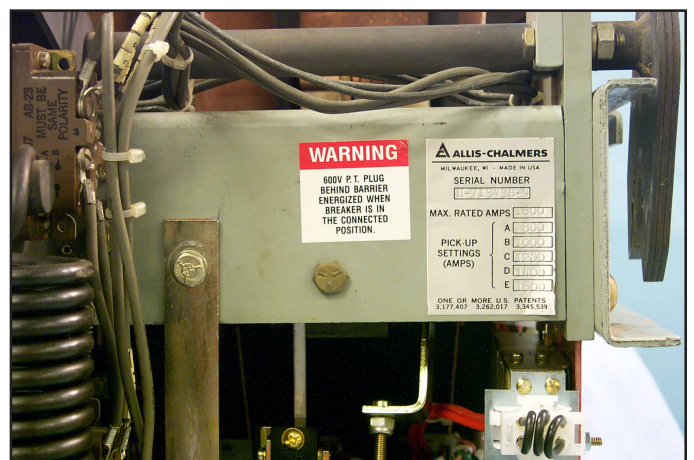
Fig. 25 PT Warning Label Installed on the Breaker.
