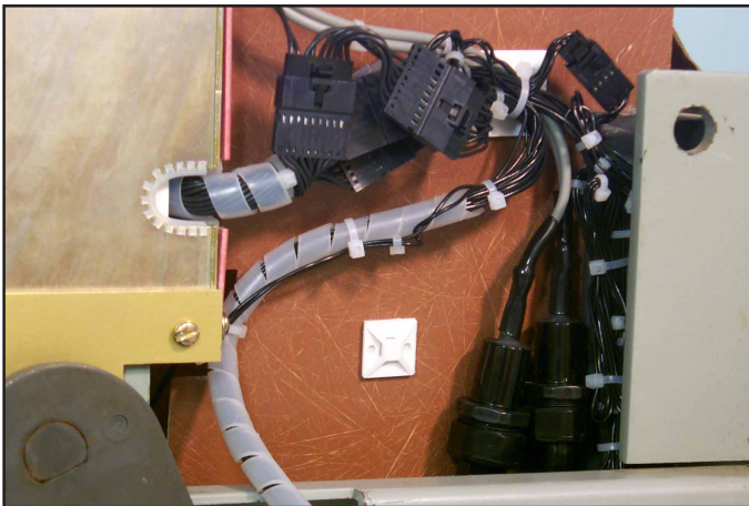
Fig. 61 HV Fuses Secured to the Breaker.
