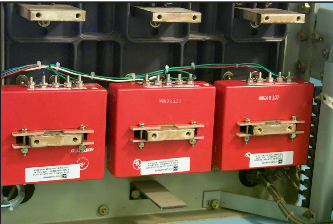
Fig. 66 Sensor Harness Connected to the Sensors.
