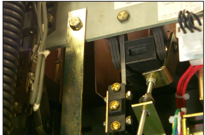
Fig. 22 Correct Positioning of the DTA Assembly Front Mounting Bracket and Auxiliary Switch Arm.
