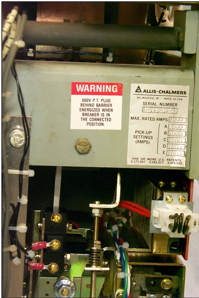
Fig. 48 Routing and Connection of the Auxiliary Switch Wires to the Auxiliary Switch.
