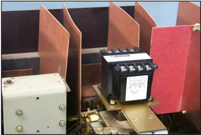
Fig. 54 CPT Assembly Installed on the Breaker.
