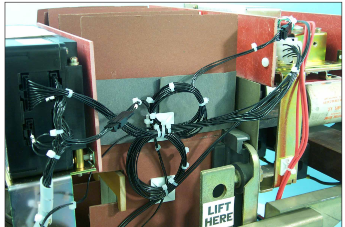
Fig. 71 CPT Harness Connected to the External Harness.
