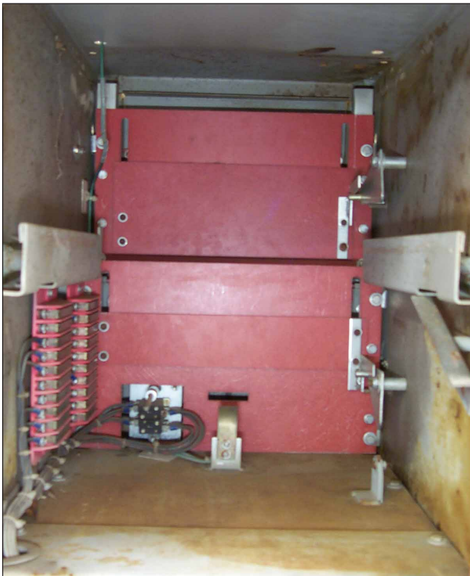
Fig. 62 The Inside of the Breaker Cell.
