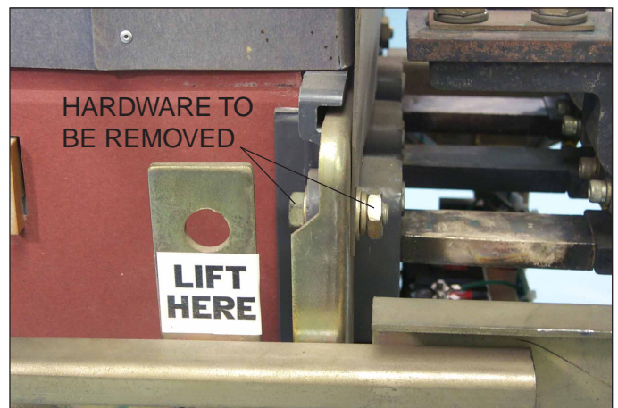
Fig. 10 Location of the Breaker Backplate Mounting Hardware.
