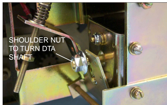
Fig. 55 Adjusting the Gap Between the DTA Trip Finger and the Trip Shaft Interlock Pin.
