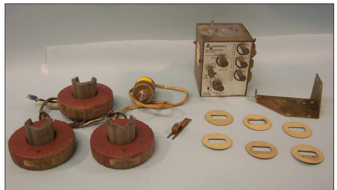
Fig. 2 Original Components Removed from the Breaker and Scrapped.
