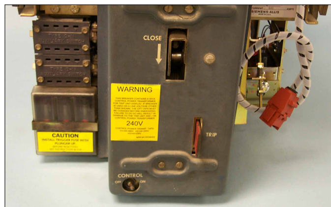
Fig. 69 CPT Voltage Label Installed on the Breaker Front Cover.
