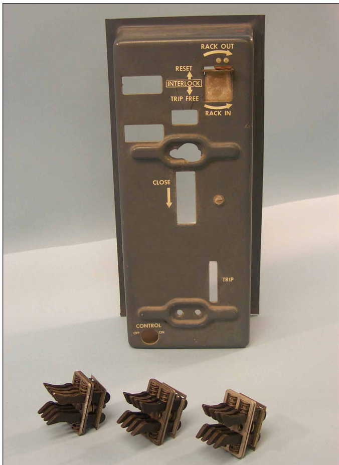
Fig. 1 Original Components Removed from the Breaker and Saved for Reinstallation.
