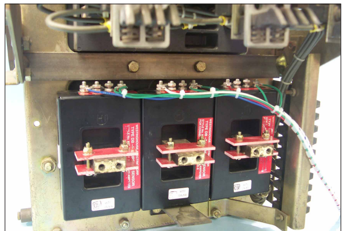
Fig. 6 Sensor Harness Connected to the Sensors.
