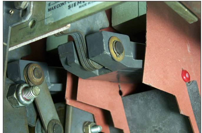
Fig. 35 Wrist Pin to be Removed from the Breaker.
