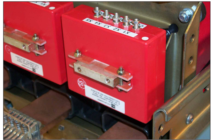
Fig. 6 Correct Positioning of the Sensors and Spacers.
