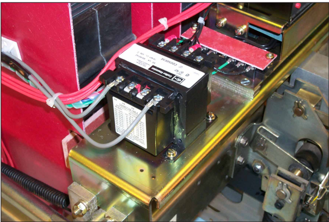
Fig. 27 HV and CPT Wires Connected to the CPT Module.
