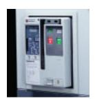
New through-the-door design provides clear and safe access to the trip unit and all breaker controls and indicators. Even breaker levering is accomplished with the door closed.
