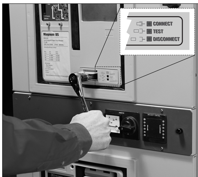
Figure 2-11 Circuit Breaker Being Levered
