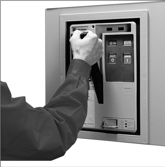
Figure 3-11 Magnum DS Circuit Breaker Closing Springs Being Manually Charged
