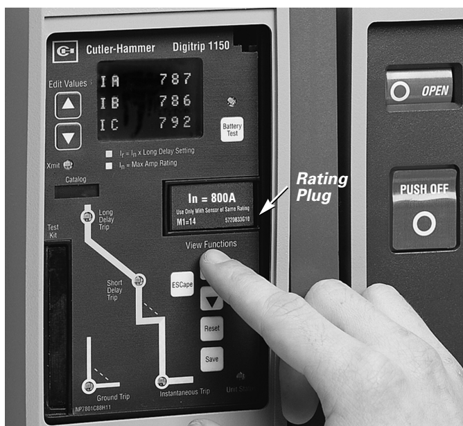
Figure 6-6 Trip Unit Rating Plug Location
