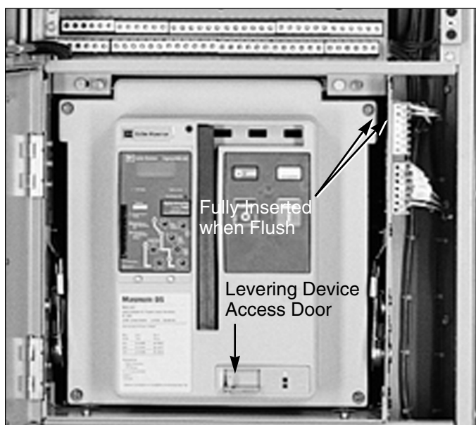
Figure 2-10 Fully Inserted Circuit Breaker
