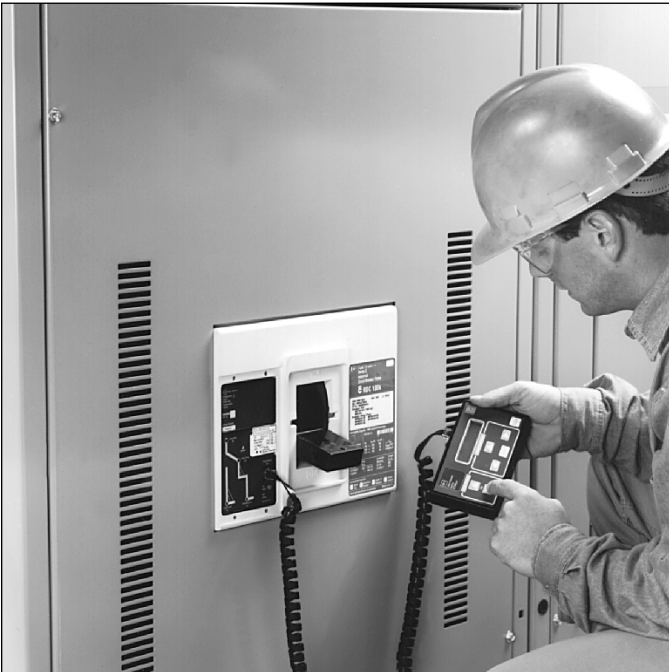
Figure 1-6 Hand Held Programmer in Use
