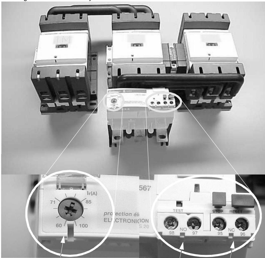
Set to minimum at the factory. Application-specific adjustment is required.
