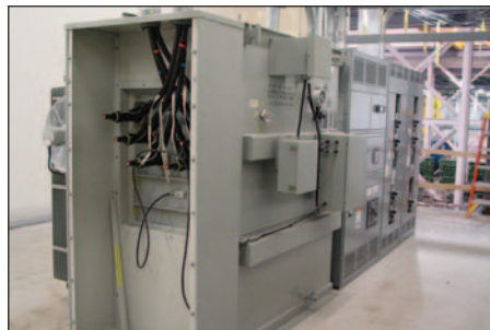
Indoor Power Center Transformer
