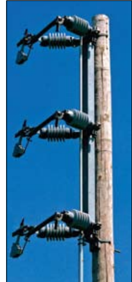
Phase-over-Phase Mounting
