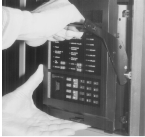
Figure 3–4: SLIDING RELAY OUT OF CASE
