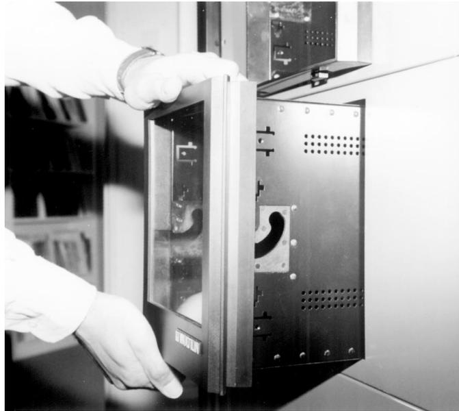
**Figure 2-3: SLIDING THE UNIT INTO THE PANEL**
